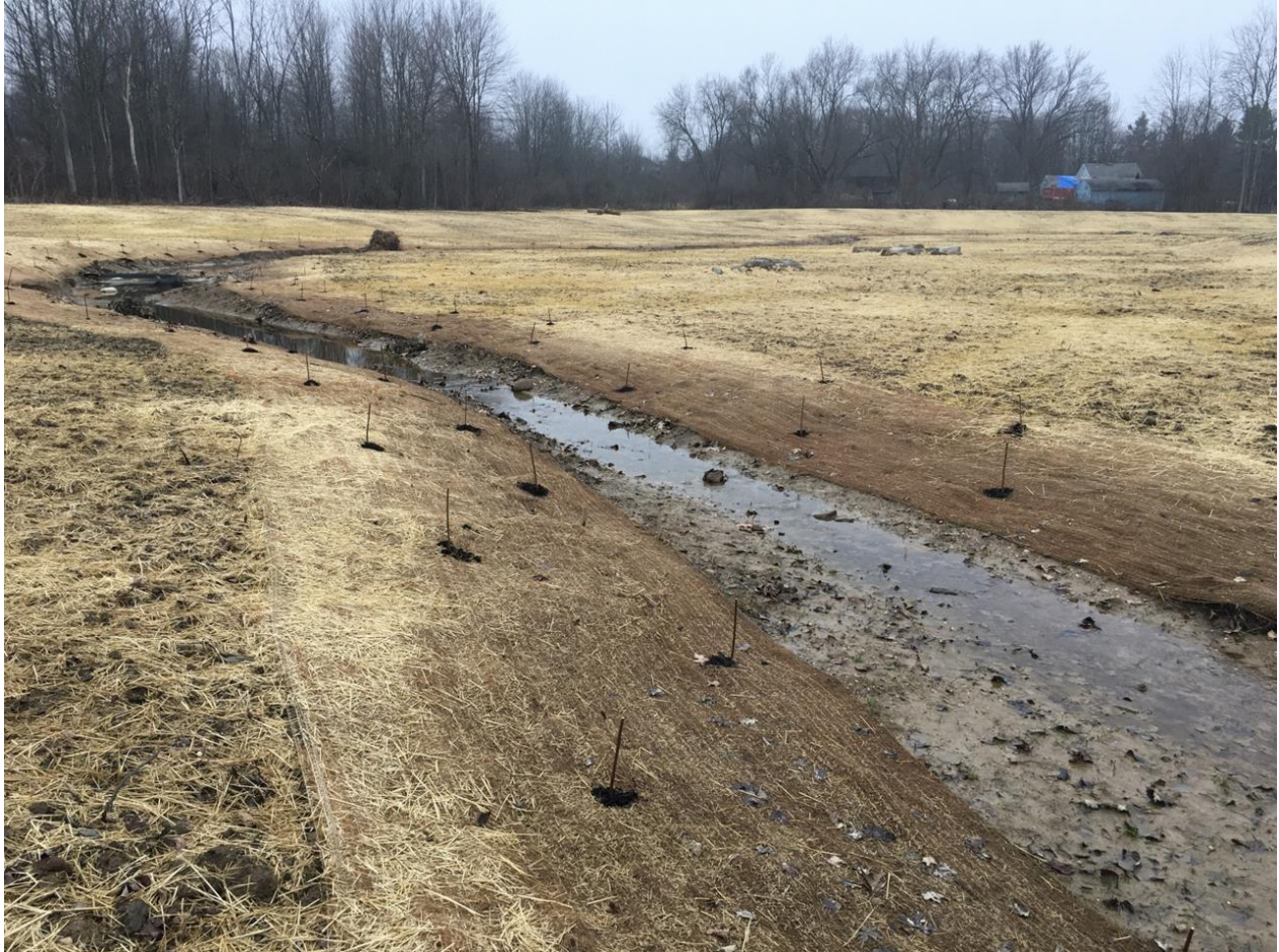
Figure 1. Facing north, after seeding, mulching, and livestock installation of the newly restored stream. Photo source: Chagrin River Watershed Partners, December 6, 2022.
