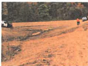
Central Retention Basin
