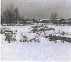
Family Life Center detention pond
